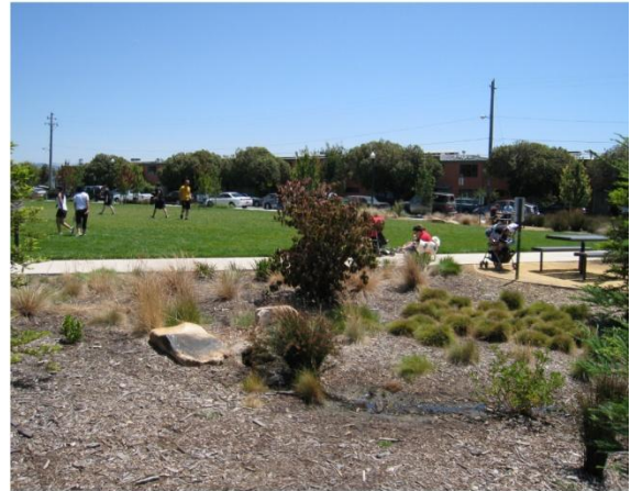
15. Sustainable Stormwater Treatment
